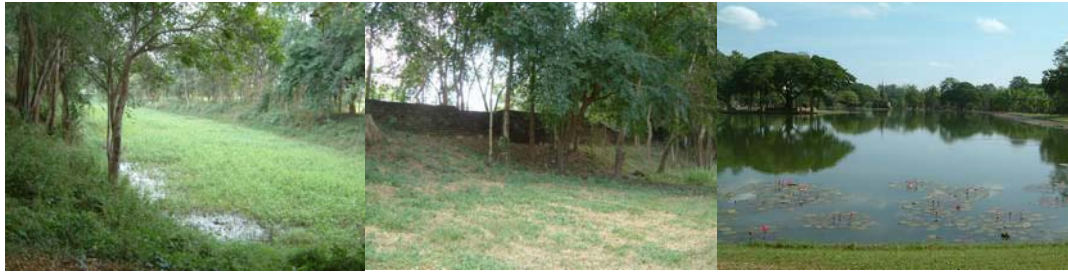
Figure 3. Existing Moat, bypass and Earth embankment of Sukhothai Kingdom.
